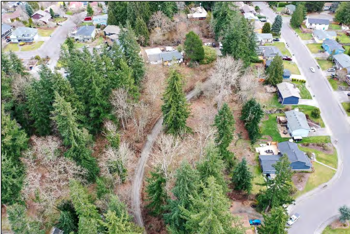
Photo 1: Overhead view of project site. Photo captured by GeoTest drone. Perspective to the east.
